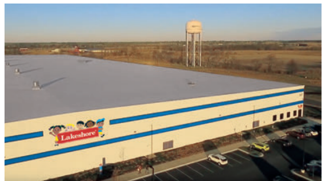
Our eastern distribution center in Midway, Kentucky.
